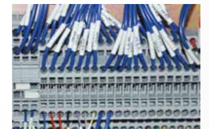
WECO connecting terminal
